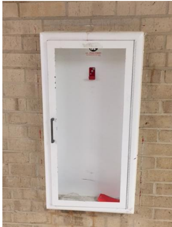
Figure 10 – Image of empty fire extinguisher cabinet on 2 nd floor at Callaway High School. There were no fire extinguishers outside classrooms on any halls. Extinguishers were placed in a closet due to students tampering with them.
