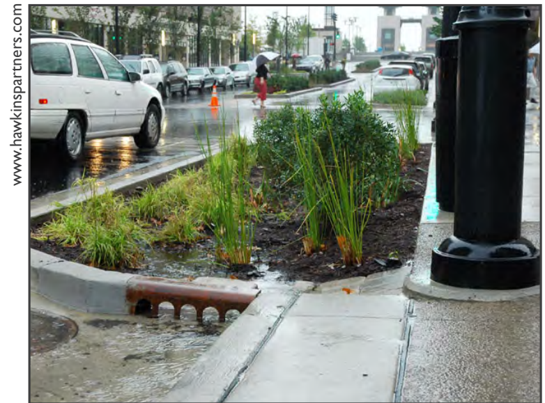
Figure 43. The rain gardens along Deaderick Street in action during a light shower.
