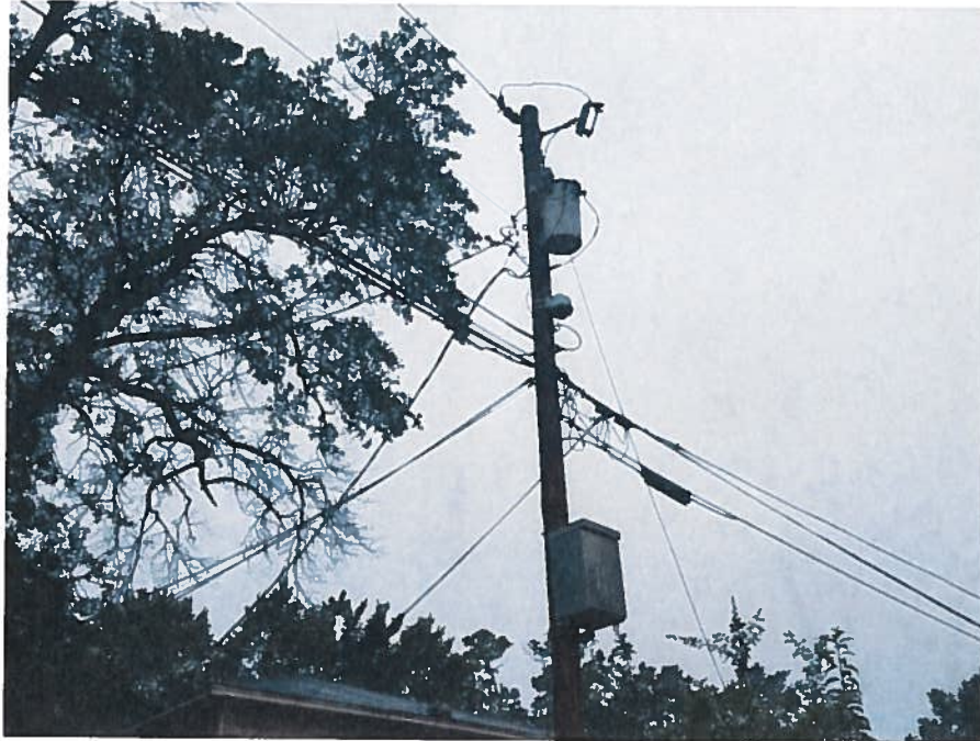
7. Pole mounted transformers along Fondren Place
